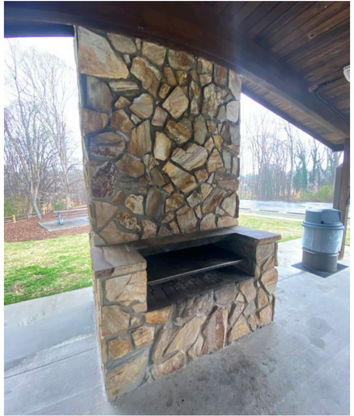
Built in fire place at the shelter
