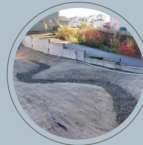
Bioswale under construction
