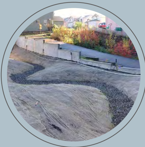
Bioswale under construction
