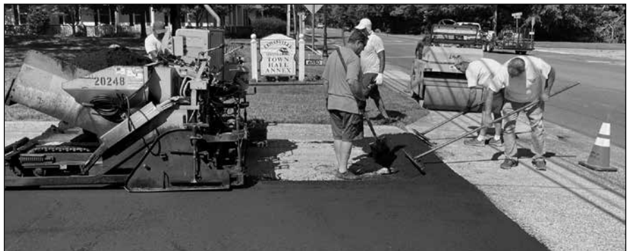
The Town Hall Annex parking lot recently received a facelift with a repaving.
